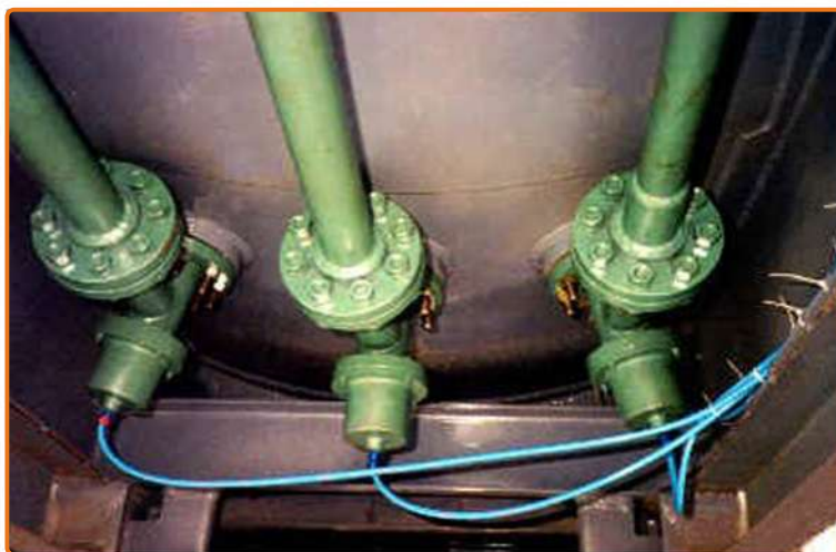
Example of VIPA F 50 assembly at the bottom of the tank.
